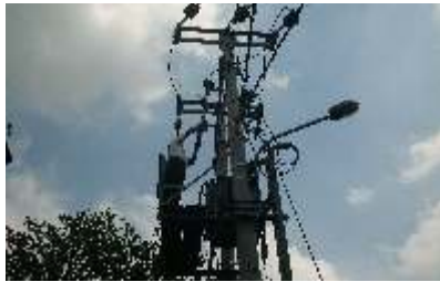
Transformer Substation
